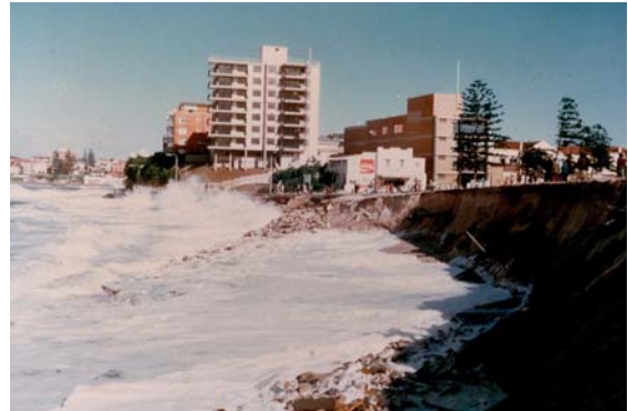
Beach erosion at Cronulla, June 1974
