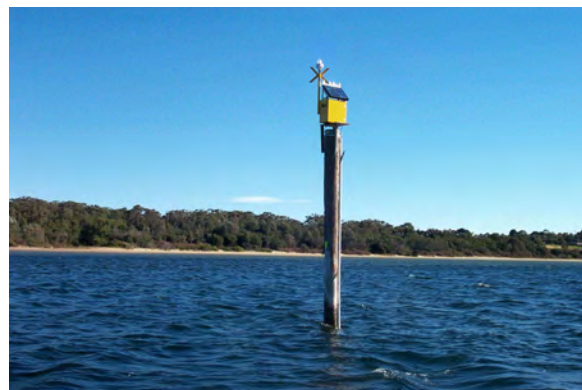
Typical tide and wave pole sensor with telemetry housing
